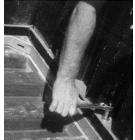
3 Vault assembles using only hand tools.
